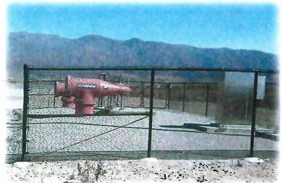
Recycled Water Line at the San Sevaine Basin #5.
